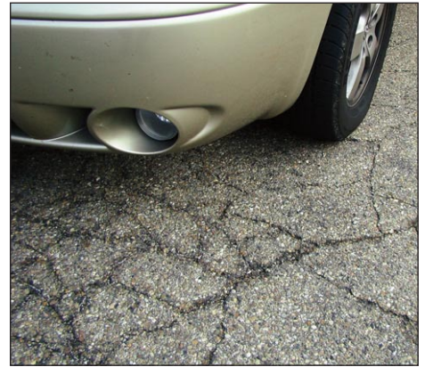
Cracking up. After ten or twelve years, the combination of wear and weather will start to fracture a road's pavement. If it is not re-surfaced at that point, the damage will extend to its sub-surface, where repairs can be much costlier.
