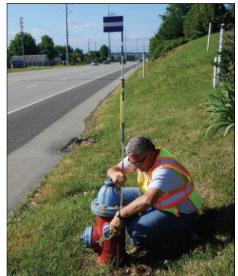
It's over here! Public Works Sewer and Water crew leader Rick Cook installs a hydrant marker along Rt. 19, making locating it easier under heavy snow.
